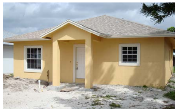
Under Construction — 2807 Saranac
