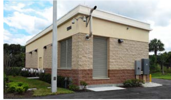
Belvedere Homes Pump Station
