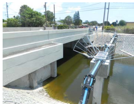
Cherry Road Bridge Expansion
