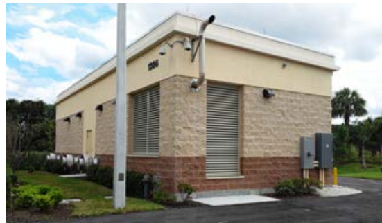
Belvedere Homes Pump Station
